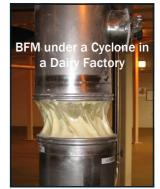
The amount of movement, environment, temperature and nature of the pressure should be taken into account when specifying a connector.
